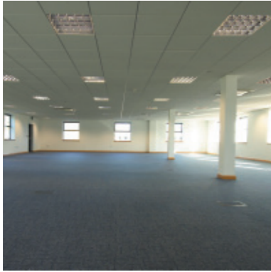
Suspended ceilings with recessed lighting.
